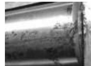
Fig. 190. Pitting on roller.
