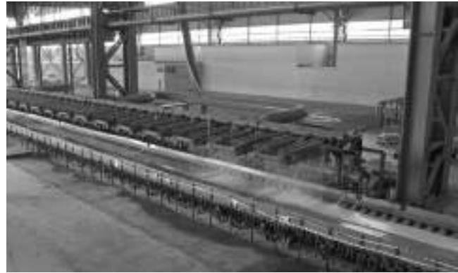
Fig. 110. Hot-strip mill roller tables.
