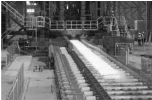
Fig. 113. Hot-strip mill transfer roller table.
