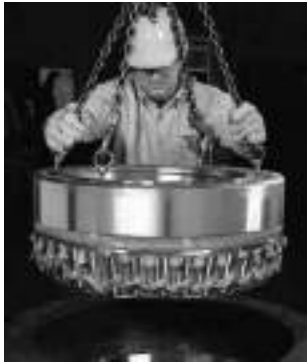
Fig. 246. Installing a greased component in the chock.
